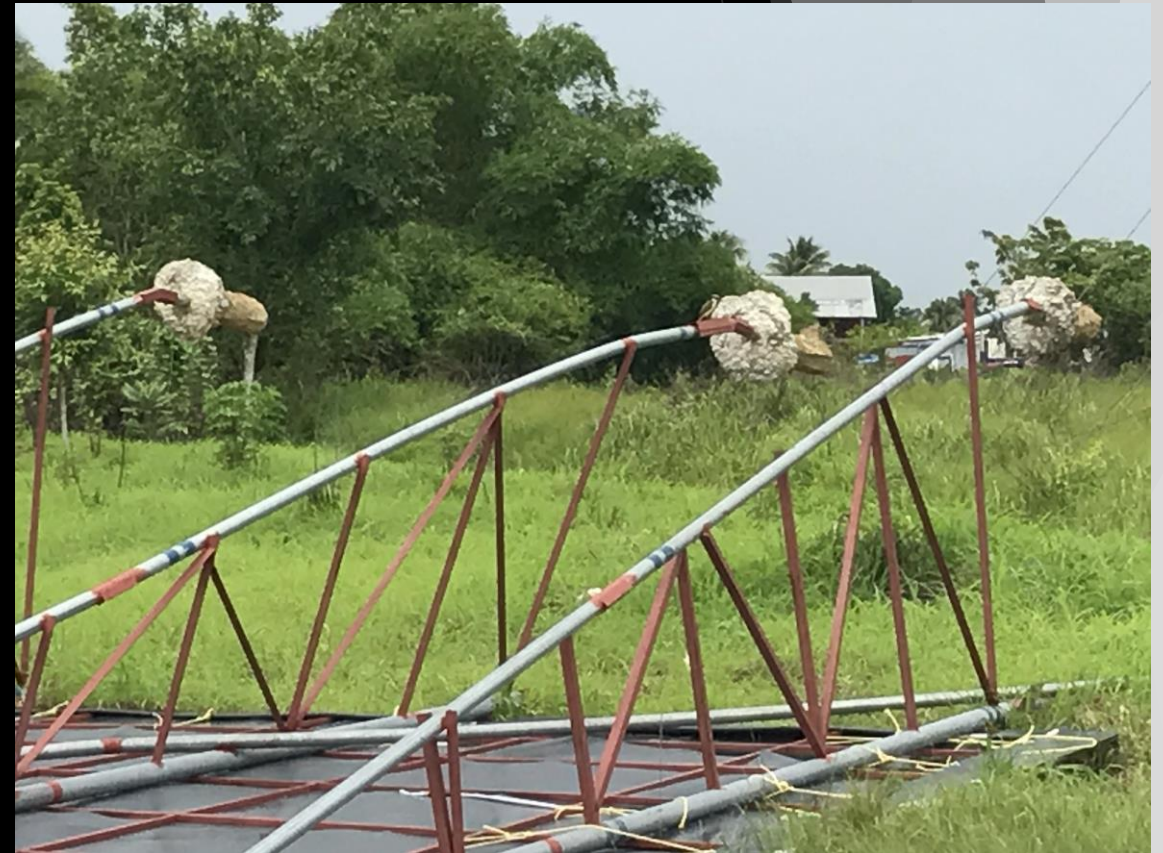
Examples of fallen billboards after the passage of Tropical Storm Bret in 2017
